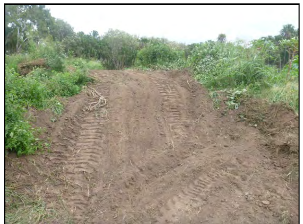
Photo 16: Stockpiles following remediation 23/04/14
