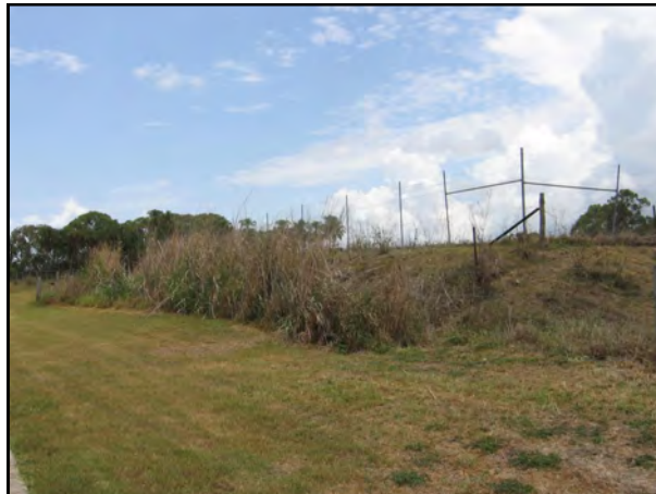
Photo 2: Northern end looking south west showing fenced area of site 12/12/09
