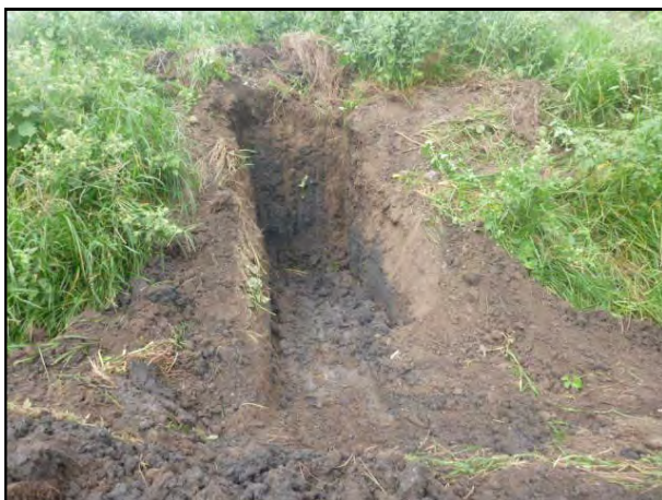
Photo 15: Test pit in stockpiles following remediation 23/04/14
