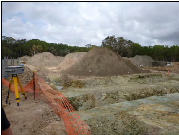
Photo 9: Excavation works looking south 24/10/11
