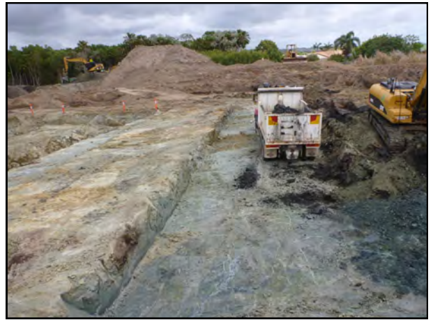
Photo 8: Excavation works looking north west 24/10/11
