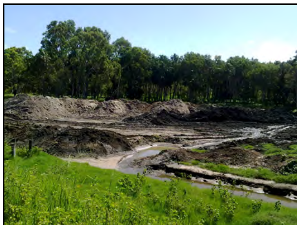
Photo 6: View of initial stockpiles to eastern portion of the site 17/02/11
