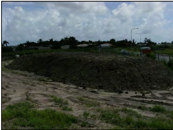
Photo 13: Stockpiles during remediation looking north 27/02/12
